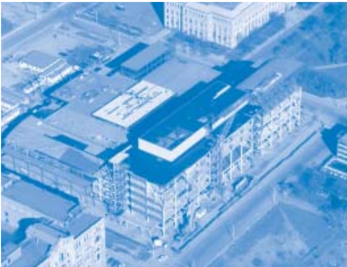
Figure 5. Aerial view of building site
