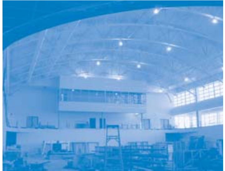
Figure 6. New gymnasium under construction
